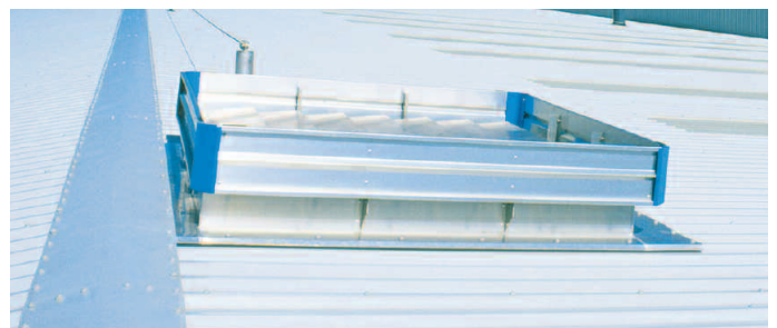
A penetration in roof cladding.
